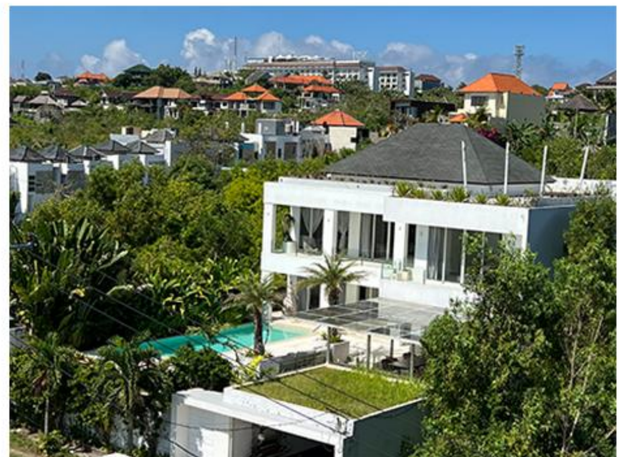
VILLA BAPAK ERY, JIMBARAN (2023) HYBRID PV 10.260 WP + BESS 12,8 KWH
